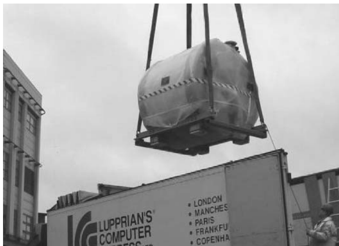
Figure 14. High Field MRI. Photograph of the new whole-body capable 3.0 tesla scanner being installed at the Centre for MR Investigations at Hull Royal Infirmary, England, one of the first of its type in the UK.
