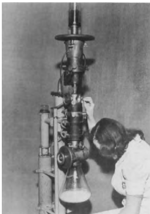
FIGURE 2. 150-kV electron microscope with image field projected onto the fluorescent material deposited on the base of an Erlenmeyer glass flask.
