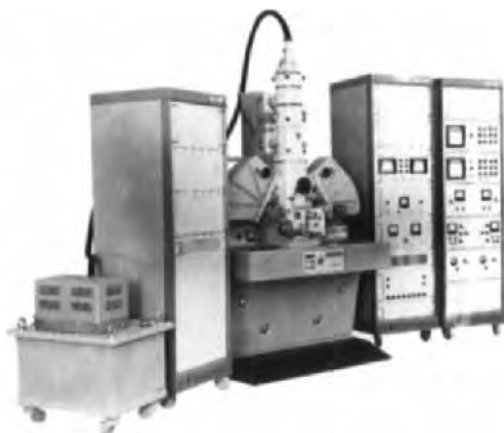
FIGURE 41. REMMA from Sumy. Based on the REMP-1, which was built in Vyborg. Its main imaging mode was by secondary electrons, and the voltage range was 10–50 kV. Elements in the range 5 to 92 were analyzable.
