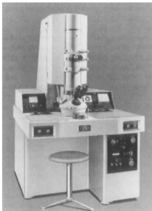
FIGURE 44. Zeiss EM 9. A very successful simplified electron microscope: 60 kV, 1.2 nm. It had automatic focusing and an automatic camera.
