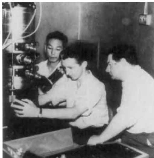
FIGURE 14. T. Mulvey (right) and M. J. Whelan (center) working with the Shimadzu Kyoto 300-kV electron microscope (1961).
