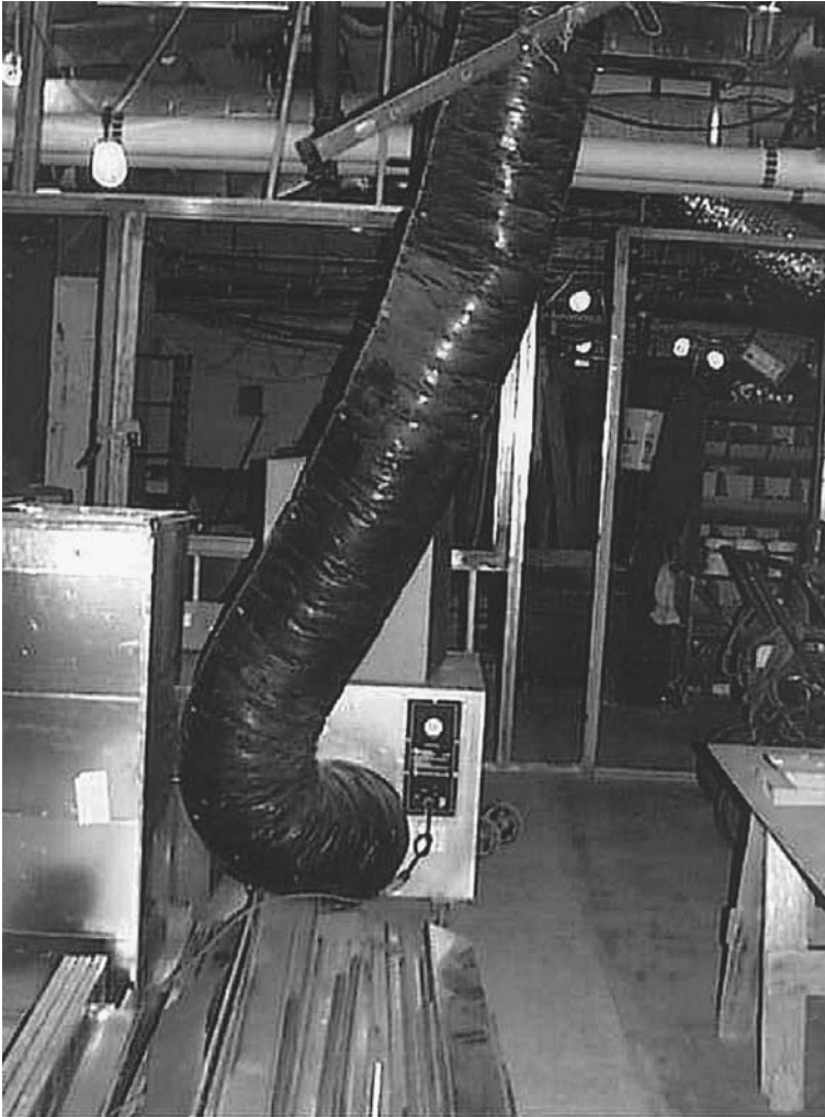
FIGURE 62.7 HEPA-filtered fan unit in construction zone used to depressurize the work-space. Exhaust is vented to building's exhaust system.
