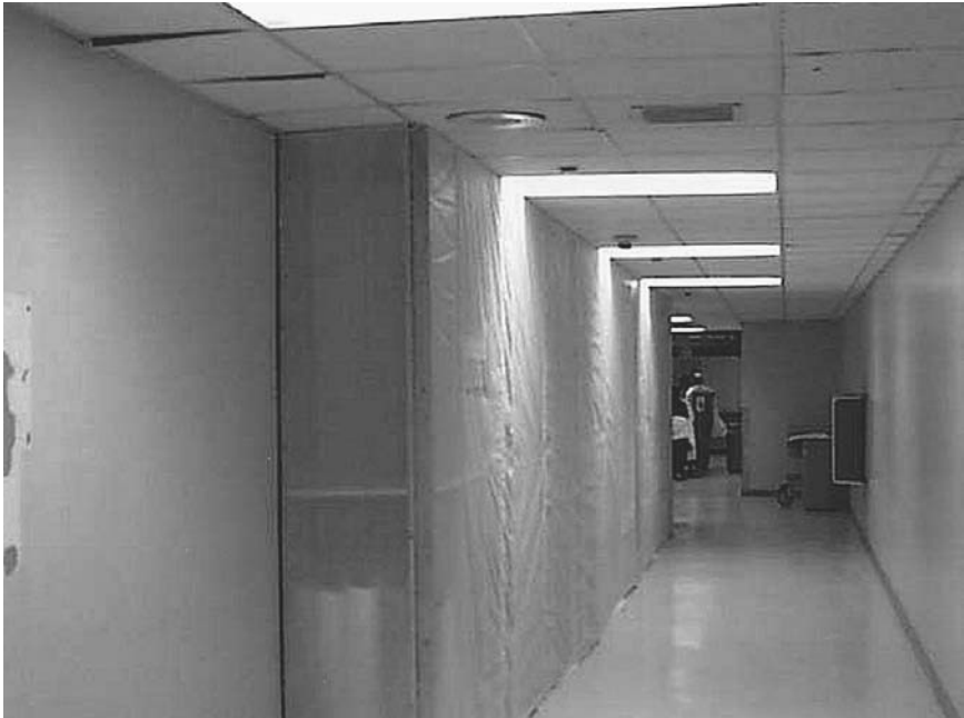
FIGURE 62.4 A temporary isolation barrier constructed of plastic sheeting and wood framing to isolate work area from occupied spaces.
