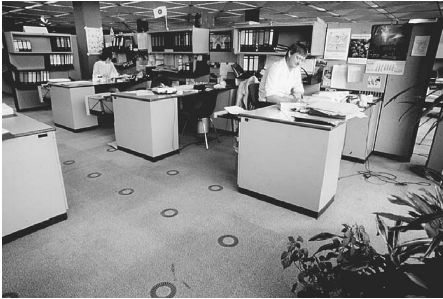
FIGURE 13.12 Balanced displacement ventilation (office). (Courtesy FGK, Germany.)
