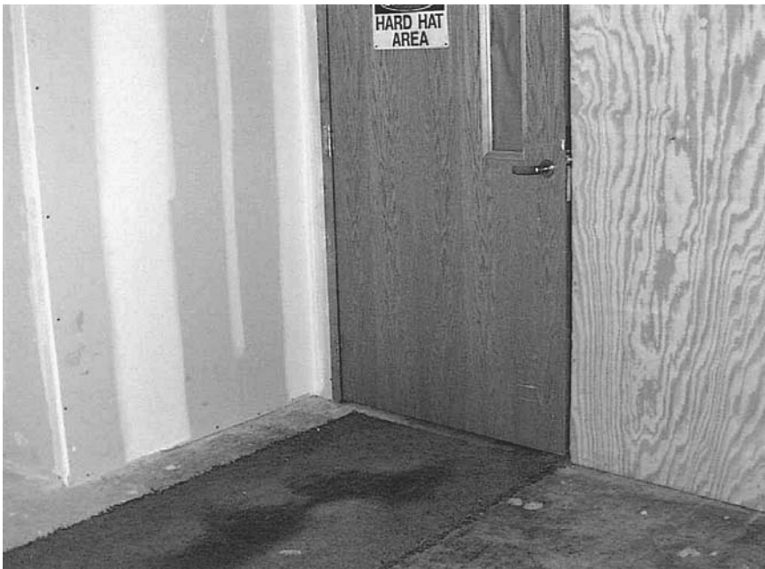
FIGURE 62.10 Temporary isolation barrier constructed of wood and plasterboard. Note use of walk-off mat. These dust control devices require maintenance, or they can be a source of dust and microbiologicals outside the contained area.
